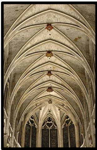
Figure 1.9. Masonry vault, Saint-Séverin Church, Paris, France [16]
