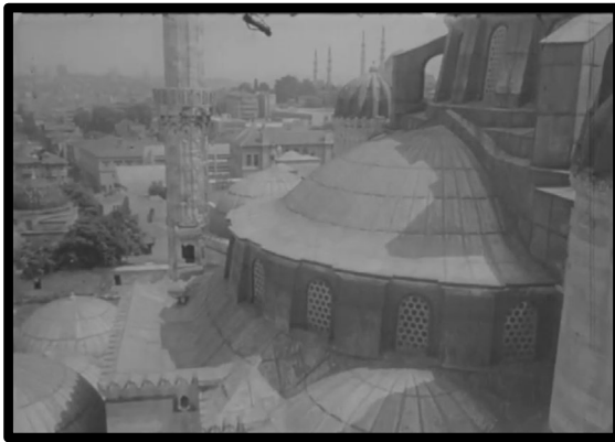
Figure 5.9. Half domes supporting the main dome [96]
