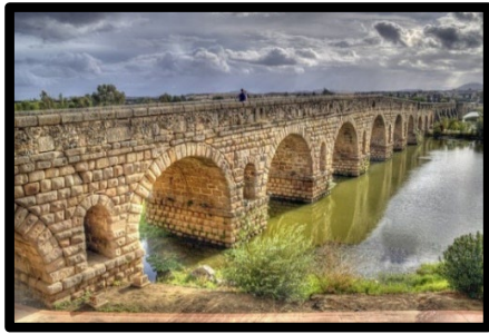
Figure 1.7. Puente romano de Mérida, a Roman bridge constructed from arches in 117 A.D. [13]
