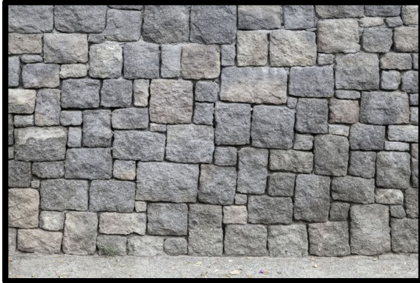
Figure 3.3. Ashlar masonry wall [55]
