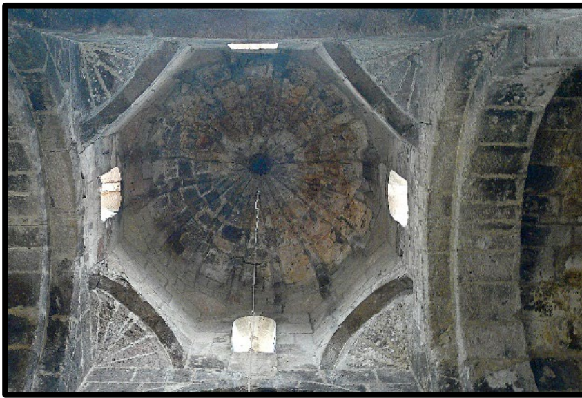
Figure 3.32. Odzun Basilica's dome, supported by 4 squinches, Armenia [82]
