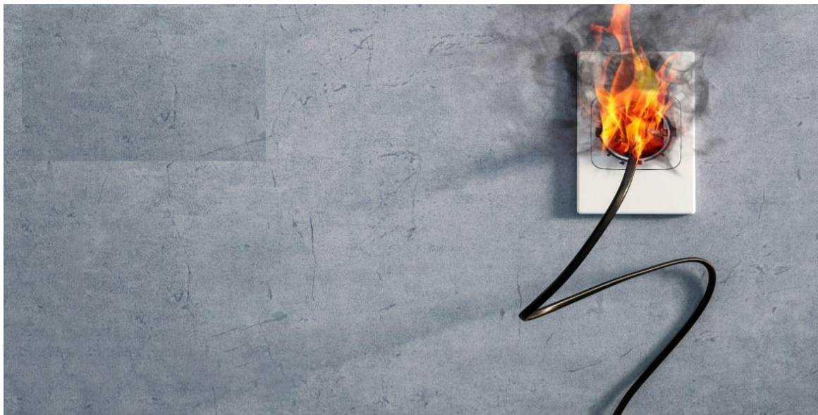
Figure 3.1. A fire caused by electricity (Campbell, 2019)
