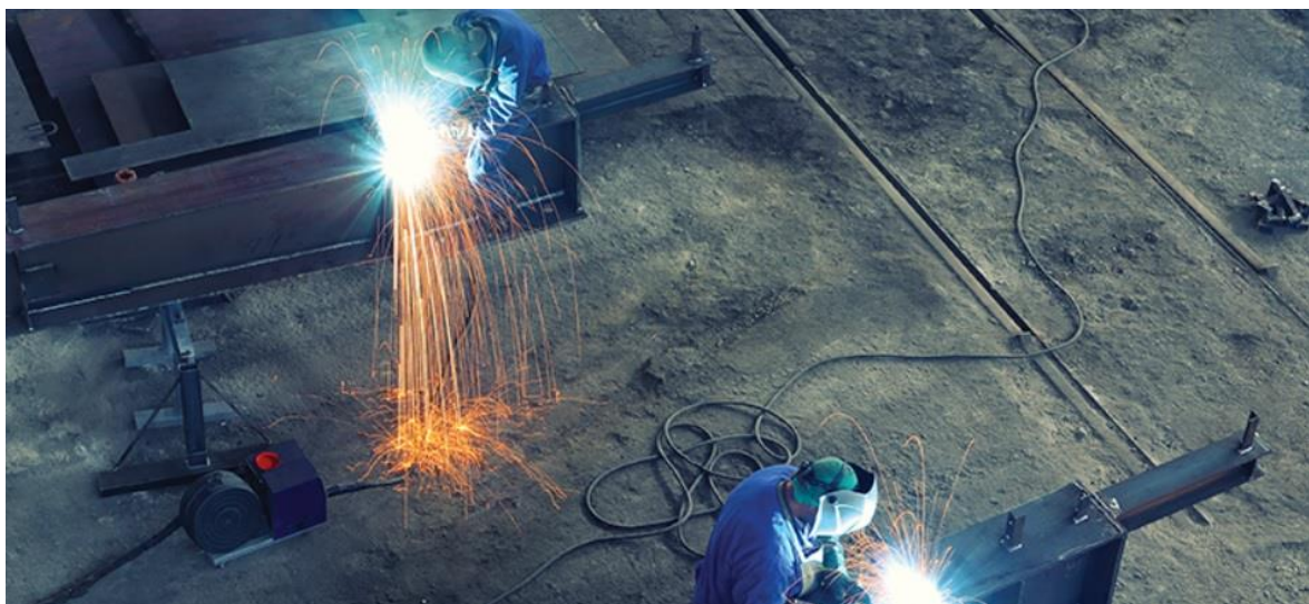
Figure 3.3. Sparkles from welding machines (Oyewole, Parasram, Shroff, and Banks, 2017)
