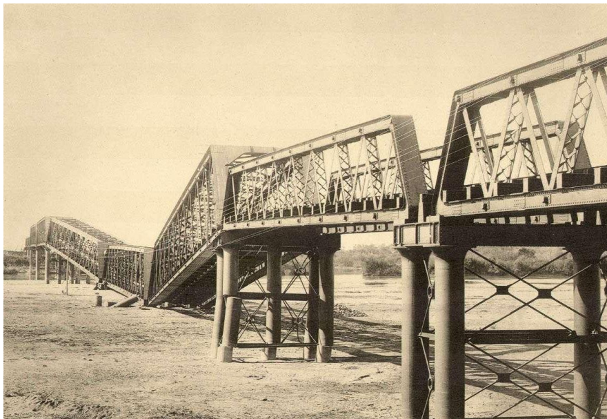
Figure 3.7. Nagara Gawa railway bridge after 1891 Nobi Earthquake (Milne, 1894)
