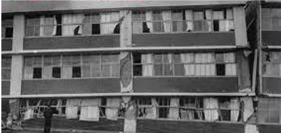
Figure 3.12. A Damage image from 1968 Tokachi-Oki Earthquake (JST, 2017).
