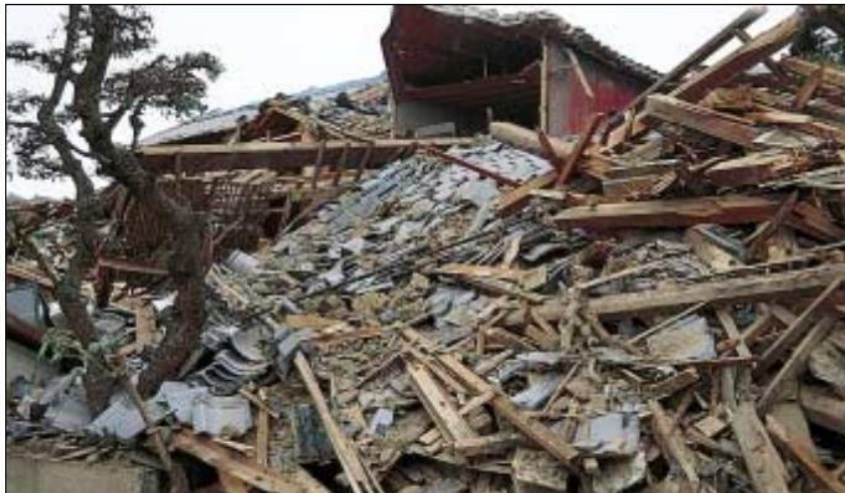
Figure 3.16. Collapsed Building in 1995 in Great Hanshin Earthquake (Holzer, 1999).
