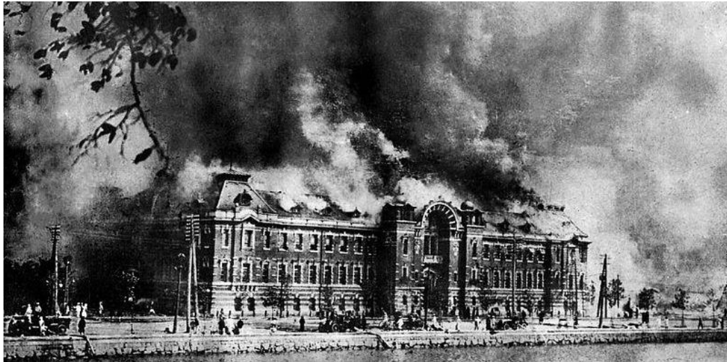
Figure 3.9. Metropolitan Police Office burning after the 1923 Great Kanto Earthquake (Wikipedia.com).
