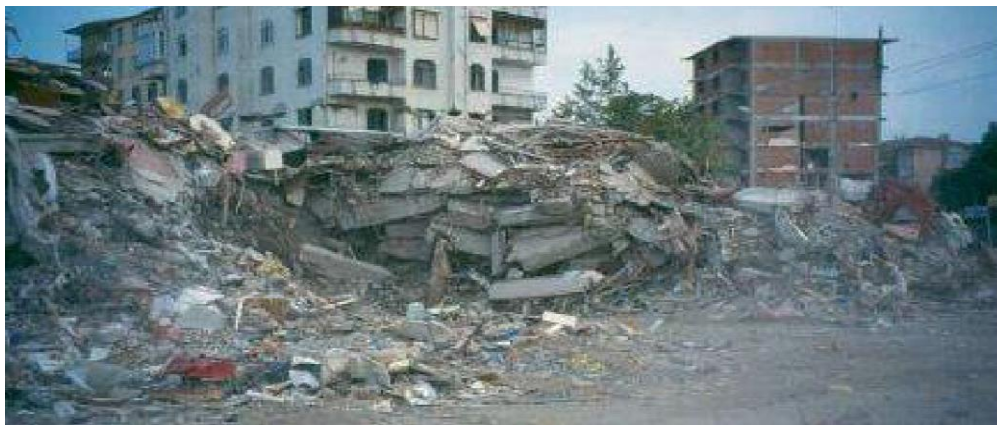
Figure 3.27. Collapsed Building in 1999 Marmara Earthquake (Karaşin ve Karaesmen, 2005).
