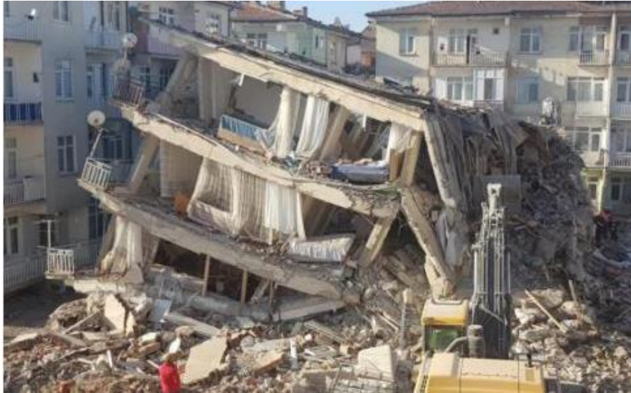
Figure 3.29. Collapsed Building in 2020 Elazığ Earthquake (Mertol, 2020).
