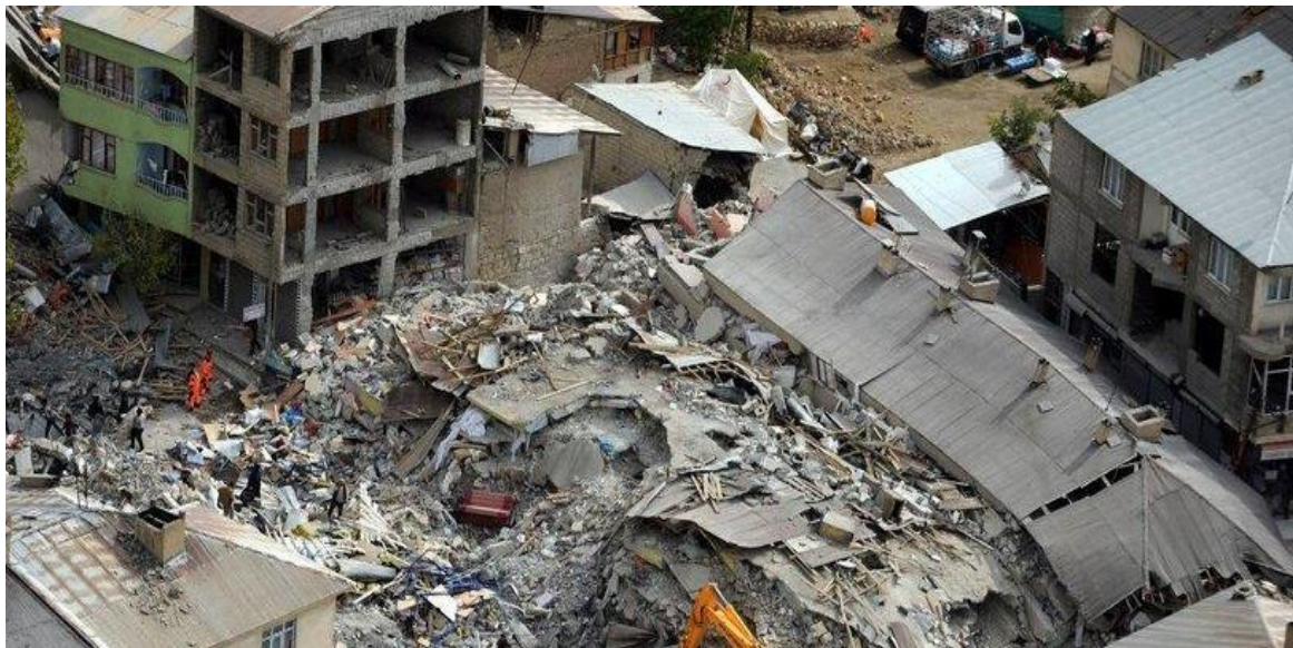
Figure 3.28. Collapsed Building in 2011 Van Earthquake (Güney, 2011).
