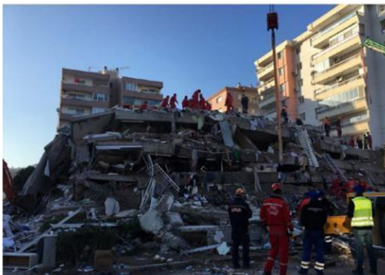
Figure 3.31. Collapsed Building in 2020 İzmir Earthquake (Deniz, 2020).
