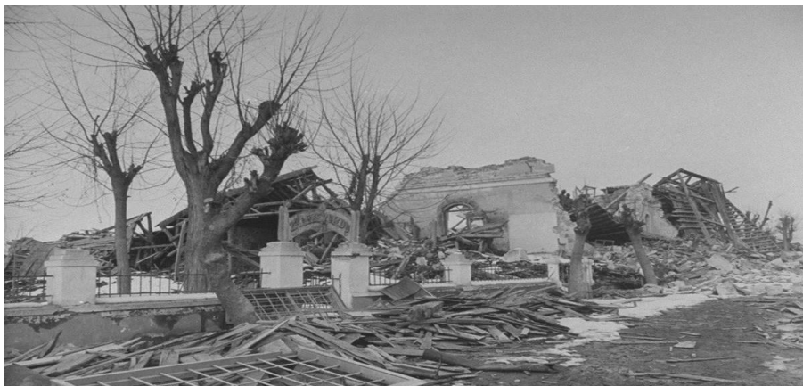
Figure 3.22. Damage from 1944 Bolu Earthquake (Bilgipedia, n.d.).
