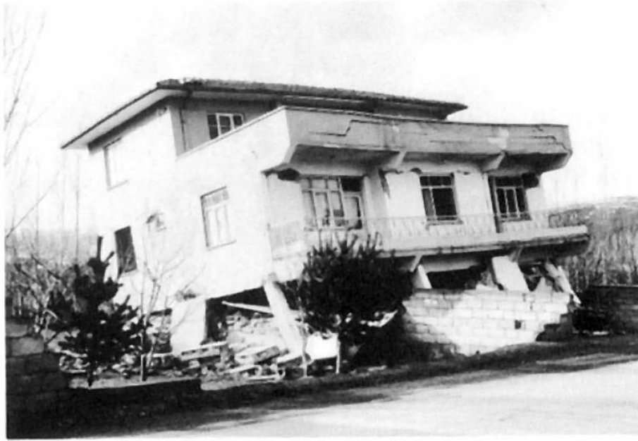
Figure 3.20. Damage from 1939 Erzincan Earthquake (William, Pomonis, Booth, & Ring, 1992).
