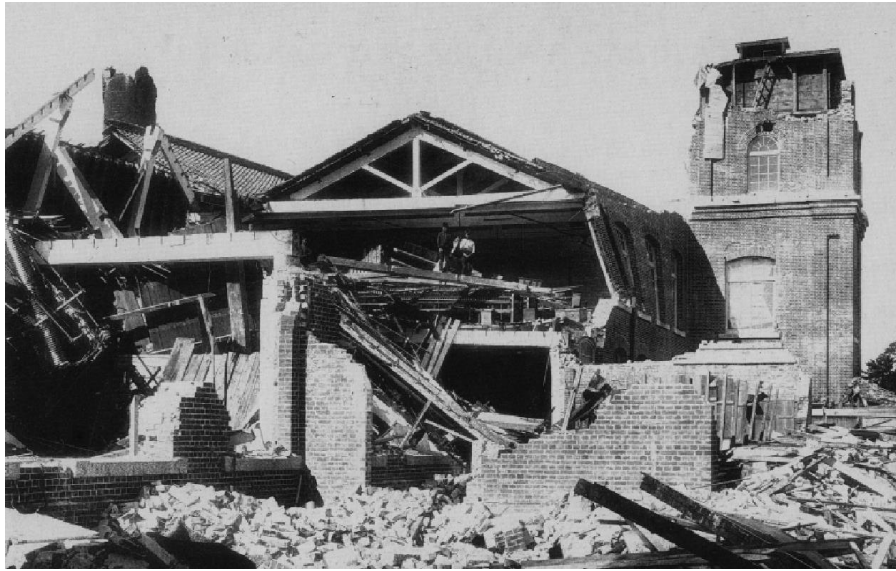
Figure 3.8. Damage of new brick factory in 1891 Nobi Earthquake (Otani, 2008)
