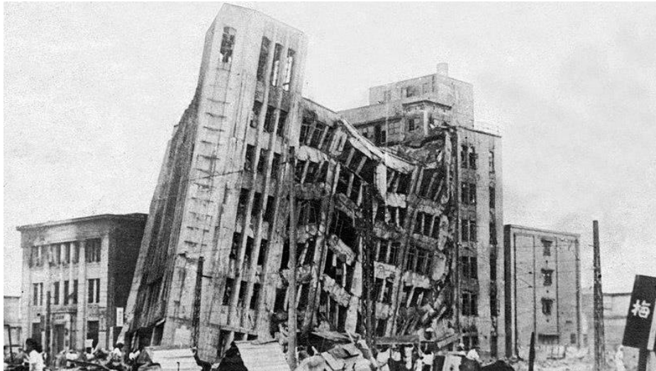
Figure 3.10. Daiwa Department Store After the Fukui Earthquake (Wikipedia.com)
