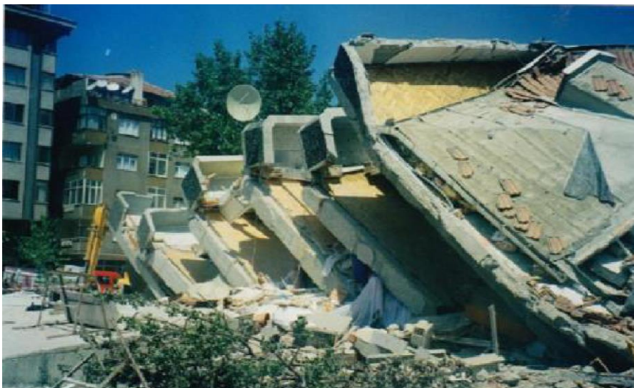
Figure 3.25. Totally Collapsed in 1999 Marmara Earthquake (Koç, 2016).
