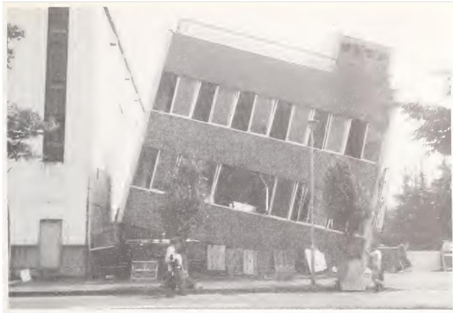
Figure 3.13. Obisan Building, Damage from 1978 Miyagi Ken Earthquake (Brady, 1980).
