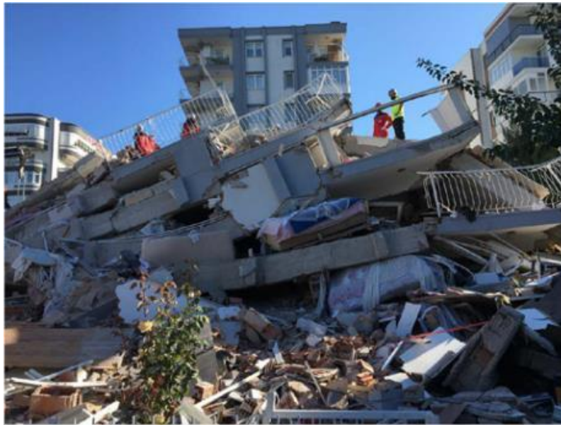
Figure 3.30. Collapsed Building in 2020 İzmir Earthquake (Deniz, 2020).
