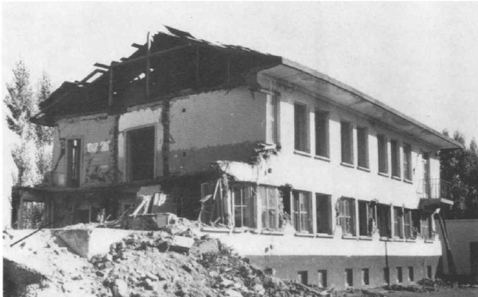
Figure 3.23. Regional Hospital Building after 1966 Varto Earthquake (Ambraseys & Zátópek, 1968).
