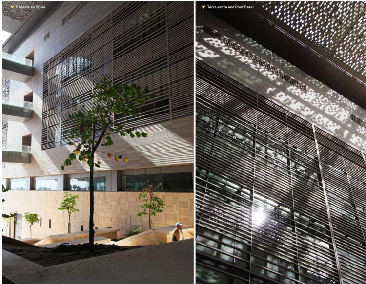
Figure 2.23. Shaded windows and skylights inspired by Mashrabiyya in KAUST (American Institute of Architects, 2010)
