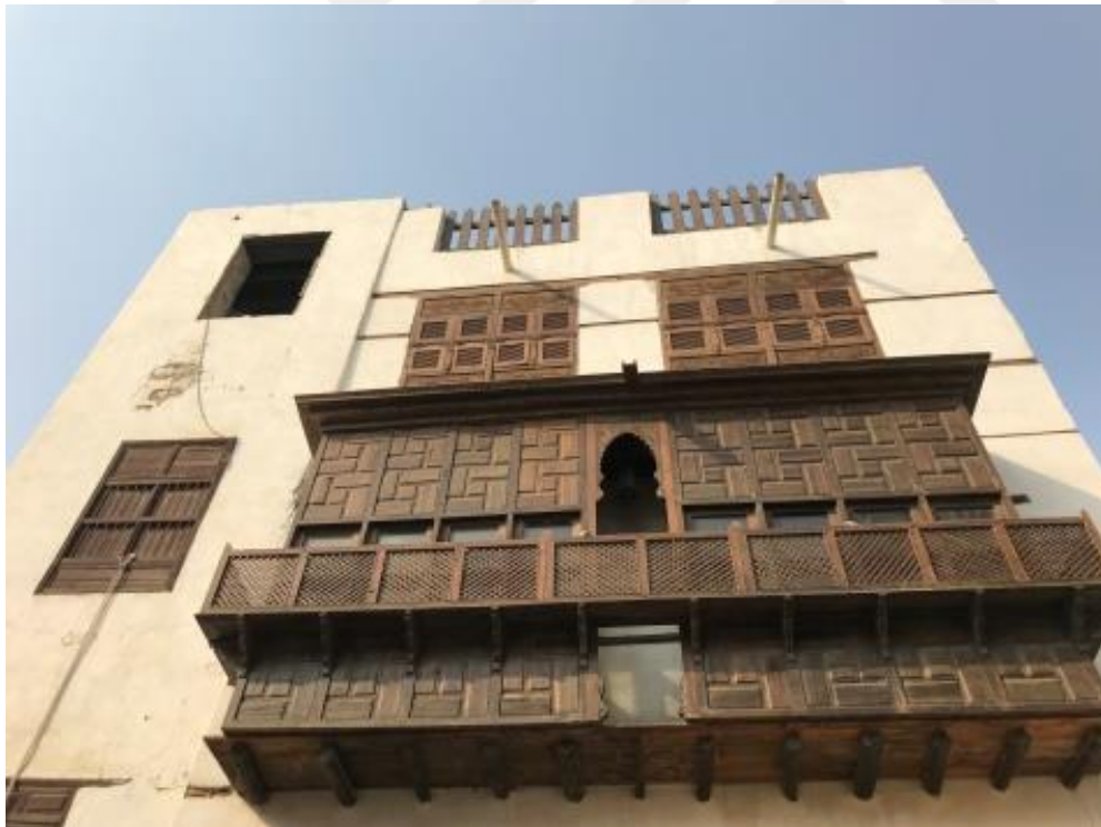
Figure 2.14. Salloum House Historic Jeddah 2018 (Nyazi's archive)
