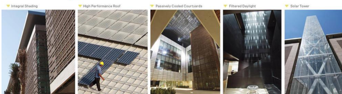
Figure 2.24. Passive design techniques in KAUST (American Institute of Architects, 2010).
