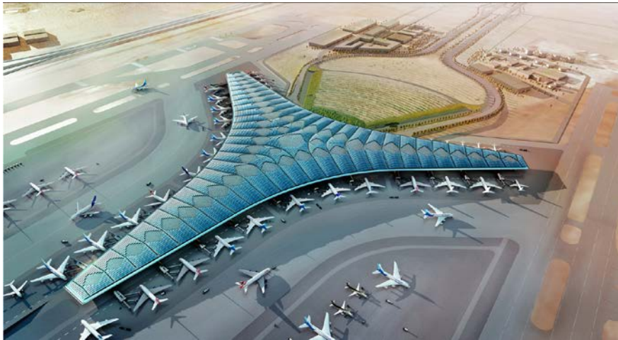
Figure 3.3. Kuwait International Airport Terminal II project
