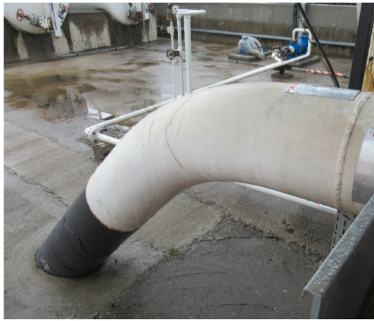
Fig. 10. Pipeline with inspection planning.
