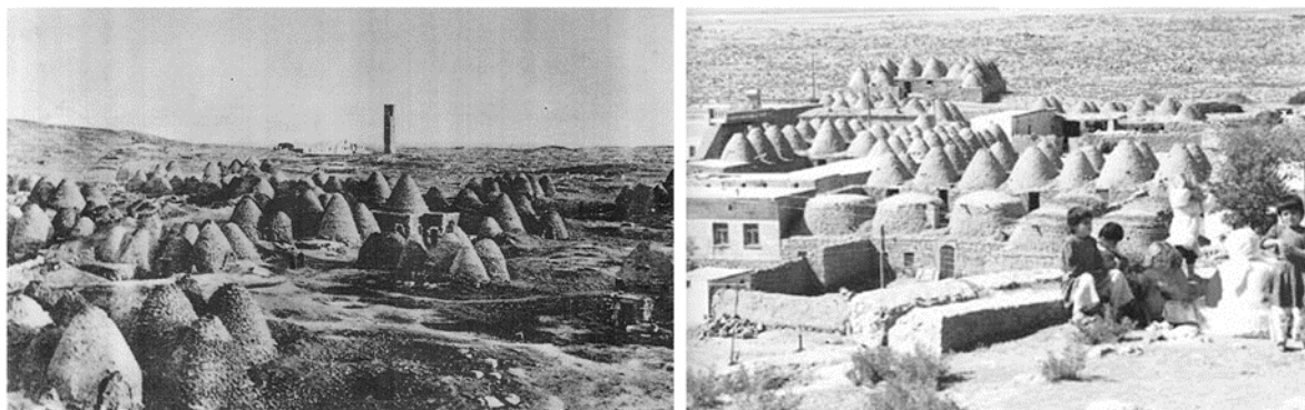
Figure 2.28. Urfa Harran Domes; in 19th century (Left) (Bekleyen et al., 1998), in 20th Century (Right) (Baran, 2006).
