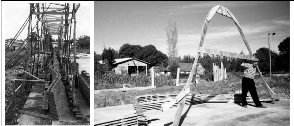
Figure 3.11. Construction of Atlantida Church (Elliott, 2019: 21-138)
