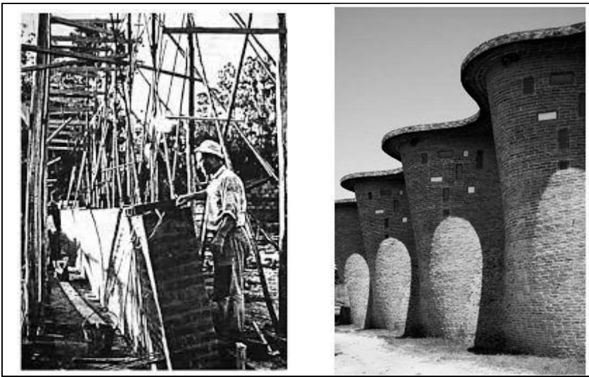
Figure 2.19. Church of Atlantida: Construction phase and built version (URL-14)
