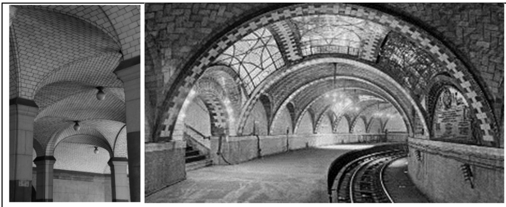
Figure 2.14. Guastavino Tiles, Manhattan Municipal Building (right) (URL-10) City Hall Subway Station, New York, 1904, by Guastavino (left) (URL-11)
