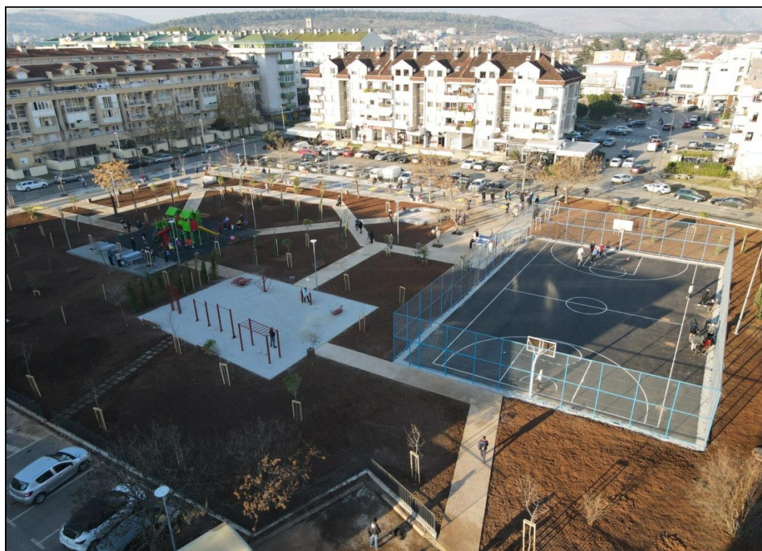
Figure 3.10. Construction of a park at the Stari Aerodrom (Source: Studio 4b, private archive)
