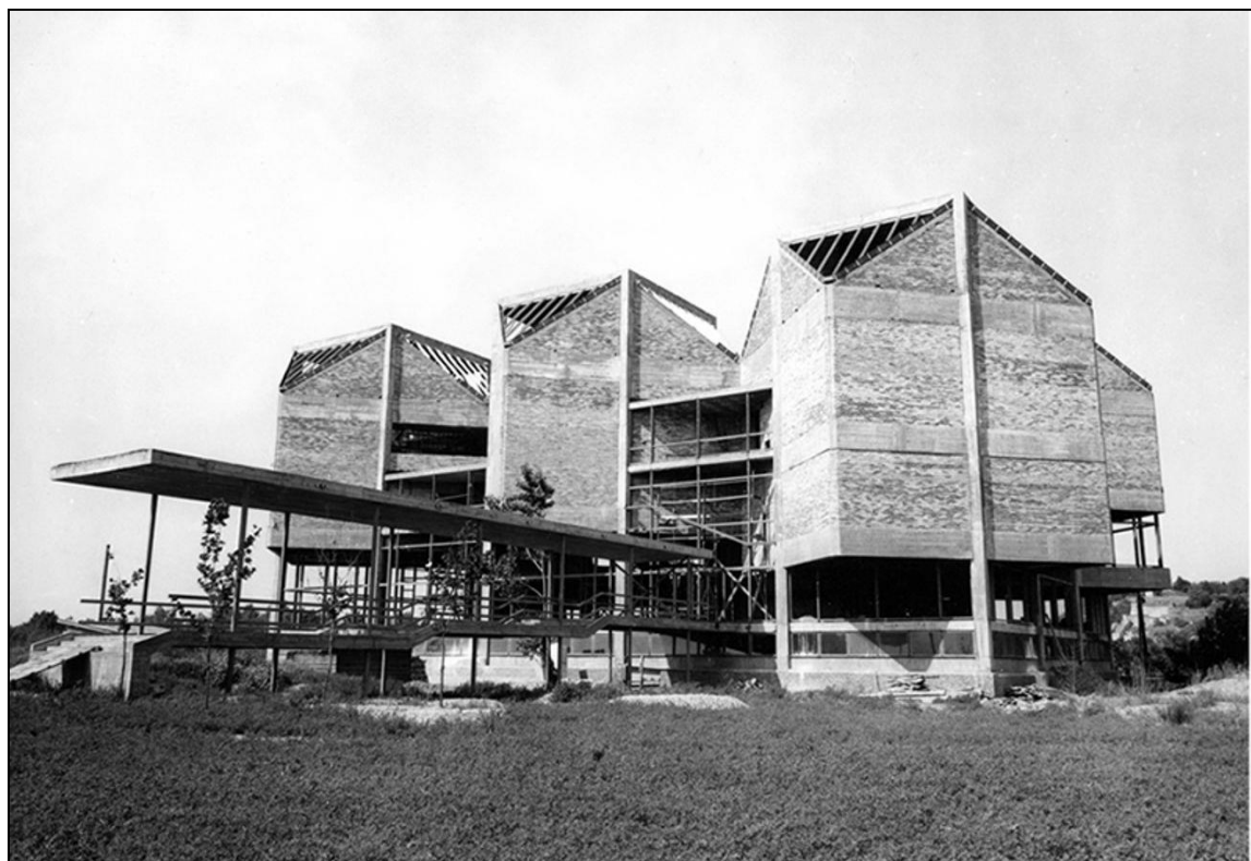
Figure 3.35. Facade during construction (Đorđević, 2017)
