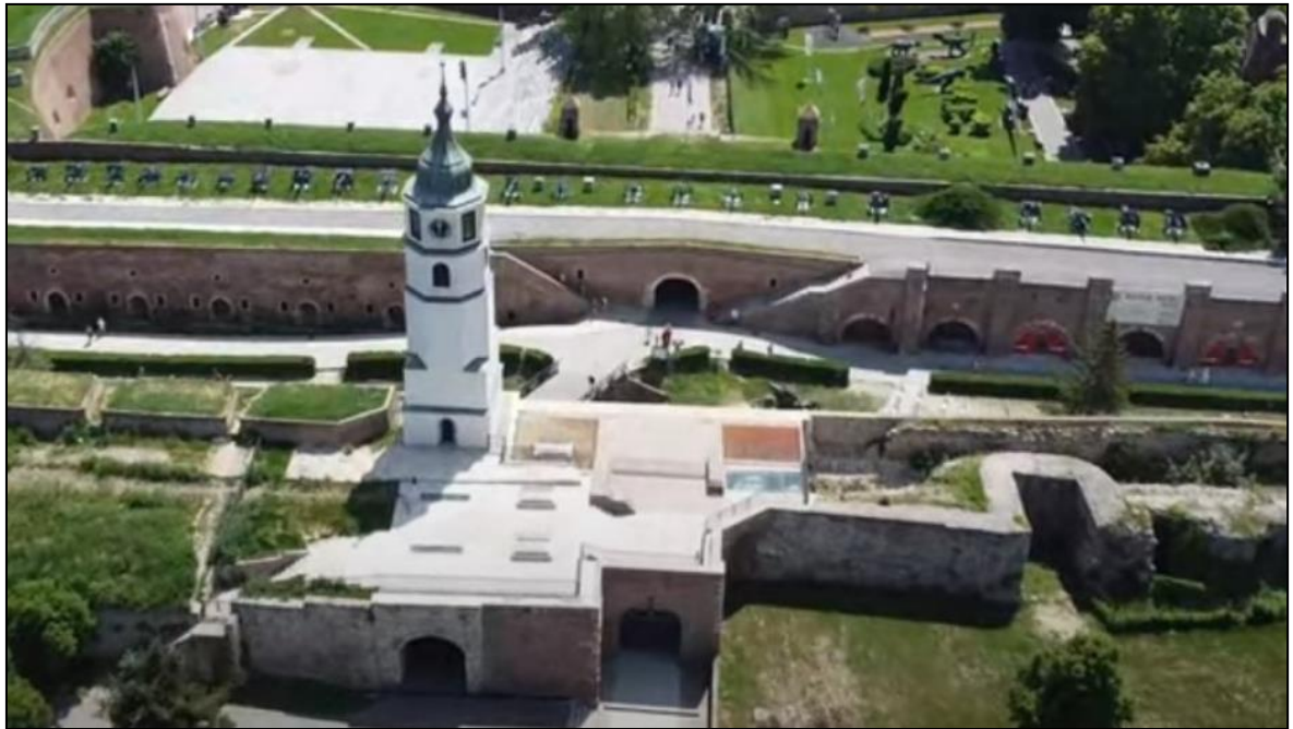
Figure 2.15. Clock tower with 3 gates today (Institute for the Protection of Cultural Monuments of the City of Belgrade. (n.d.)
