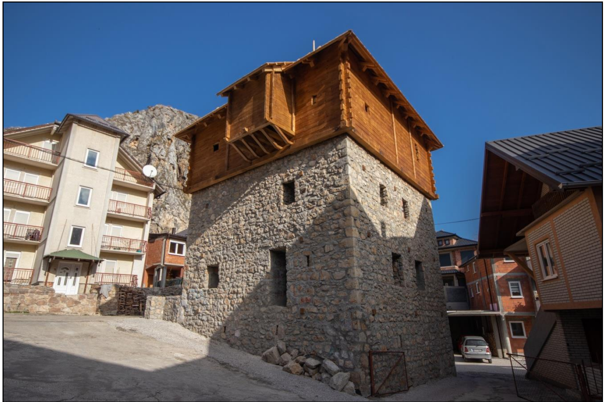
Figure 2.19. Renovated facade, Ganića Tower(Euro Projekt)
