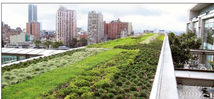
Image 2.37. Extensive green roof (URL-73)
