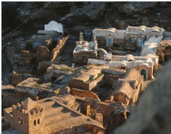
Image 2.14. Dwellings in Zriba Olia village covered with vaulted roofs (URL-48)
