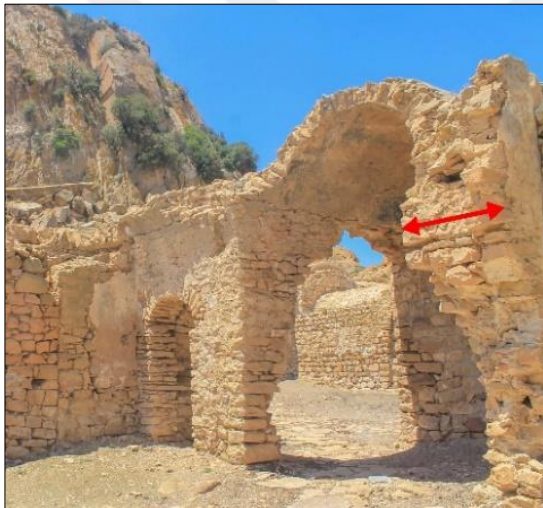
Image 2.13. A picture showing the wall thickness in a ruined dwelling in Zriba Olia village (URL-47)
