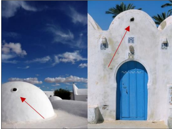
Image 2.22. Air vents placed in the vaults and domes of a Djerbian house
