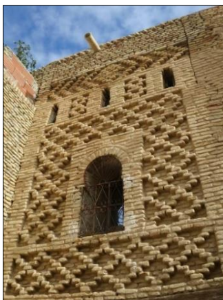
Image 2.19. Brick cladding in a house façade in Nafta (URL-52)
