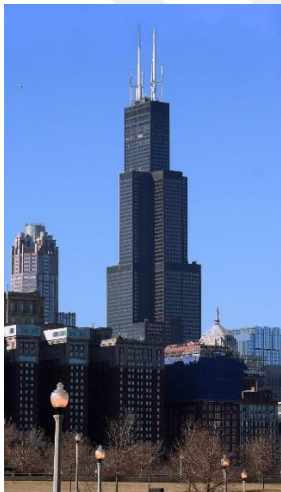
Resim 3.14. Chicago, Sears Towers Building (1974) [61]
