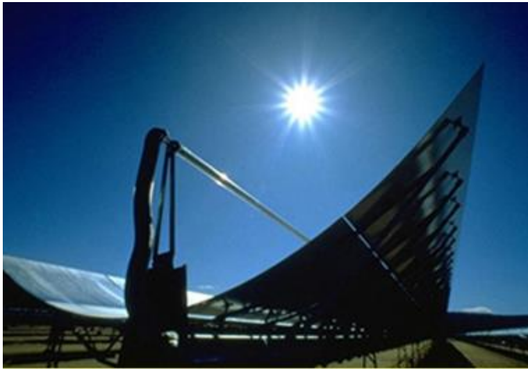
Figure 1.1. Image of trough system
