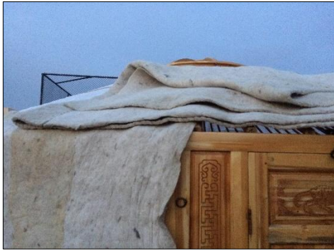
Figure 3.16. Roof covering
