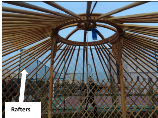
Figure 3.12. Structure of rafters
