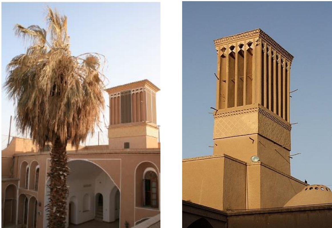
Figure 5.12. Traditional Wind Catcher in hot and arid area, Yazd, Iran (Narguess, 2009)
