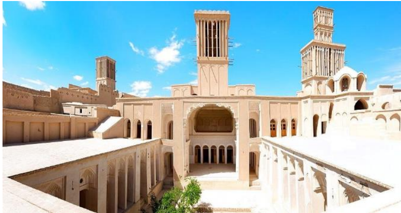
Figure 5.43. wind catcher and courtyard (Internet: G&M Therin-Weise, 2019)
