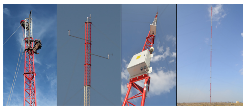
Figure 3. Installation works of the wind measurement station.
