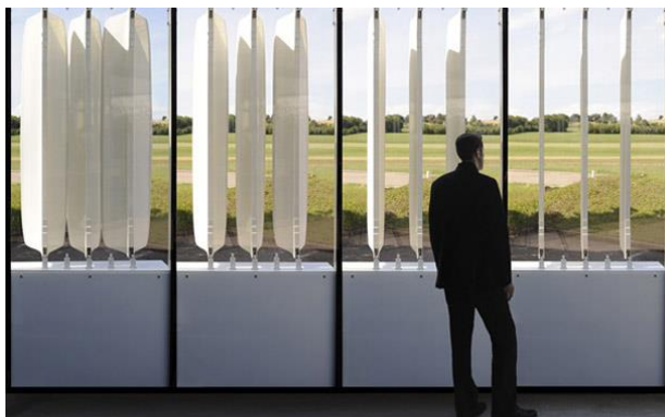
Figure 3.19. Adaptive architectural envelopes: Flectofin(López, Rubio, Martín, & Croxford, 2017)
