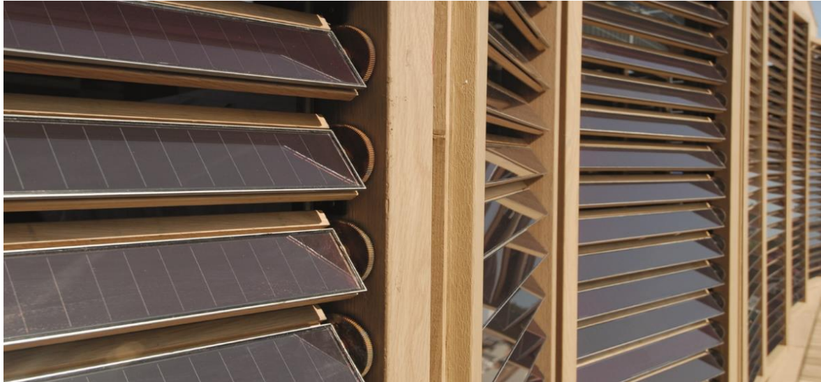
Figure 3.5. Intelligent façade of automated wood louvers (Velikov & Thün, 2013)
