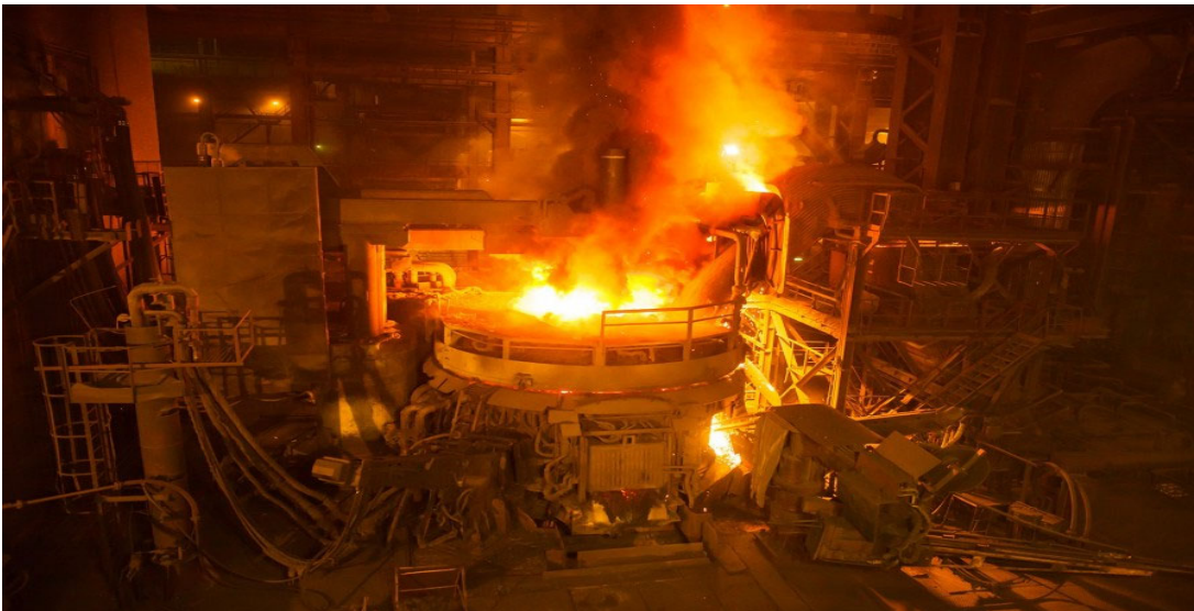
Figure 2.1. A 135 tons capacity and 180-MVA EAF [21].
