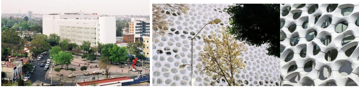
Figure 2.12. The Torre de Especialidades The smog fighting façade (Wolfson, 2013)
